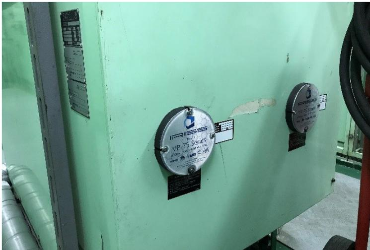
The above photo shows a dry step-down transformer with the VPT-75 installed.
