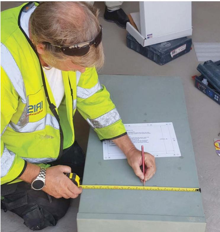
Figure 1 Paul Goodbody of IRISS demonstrates how to utilize an IR window template
