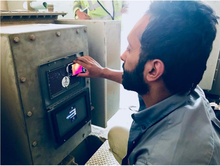
Figure 2 SEC Engineer performs an infrared inspection on a transformer cable compartment using a CAT S60 Phone with built in IR camera and a CAP-ENV-12-PD Inspection Window
