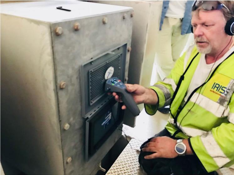
Figure 2 Paul Goodbody of IRISS listens to the Airborne Ultrasound signature on the MV side of a transformer using a SONUS PD handheld Partial Discharge detector
