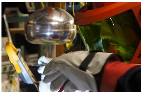
In short, the best way to reduce risk is to eliminate it. This is why NFPA 70E and OSHA state very plainly that electrical equipment should be de-energized prior to opening. Realizing that this is not always possible for troubleshooting, inspecting or in situations where shutting down is not viable or poses a risk, there is an allowance made for PPE to be used as a last resort – similar to the least preferred method in the hierarchy of control.
